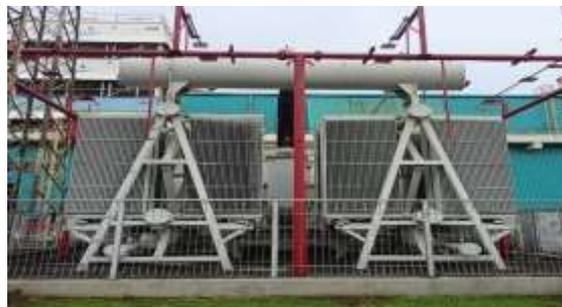
Gambar 3.1 Transformator Daya PLTGU Muara Tawar
